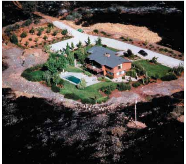
The pre-fire activities implemented by this homeowner included a green and well maintained landscape, reduction of wildland vegetation around the perimeter of the property, a fire resistant roof, and a good access road with a turnaround area. The charred surroundings of the home show that these pre-fire activities effectively protected it when wildfire hit.
